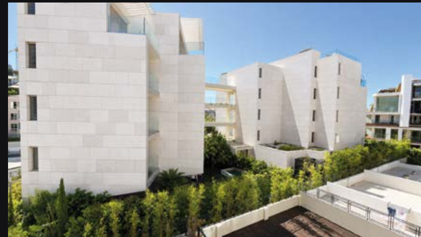
rear balcony view
